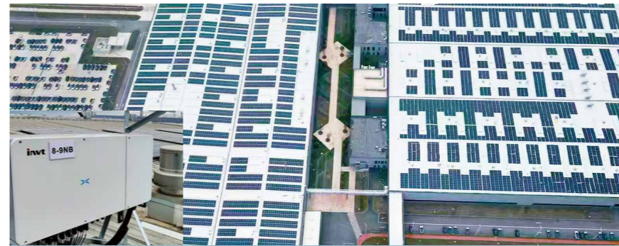
5.99MW ENOVATE Motors EV Manufacturing Base PV Plant in Changsha, China (XG110KTR, XG50KTR)
