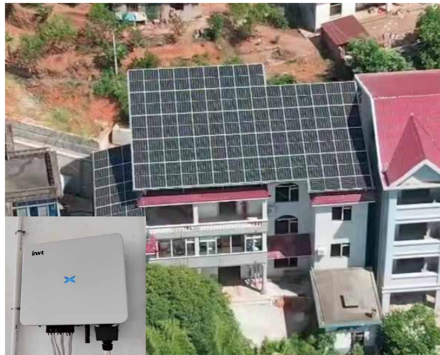
40kW Solar System in Jiangxi, China (XG40KTR)
