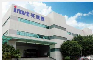
Shenzhen Fuyong Industrial Park
